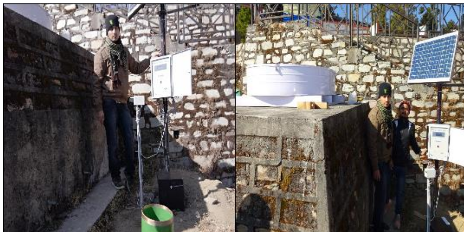
AWS installed at Gurudabaj
